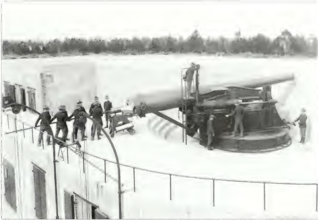
Figure 4.10. View looking northeast at emplacement #1, Battery Granger, 1899. A raised platform on the gun carriage allowed an artillery officer views over the concrete structure to a potential target. Although the gun carriages are not extant, views from a comparable vantage point and from the battery commander's stations are presently obstructed by large woody vegetation (GATE 7778).
